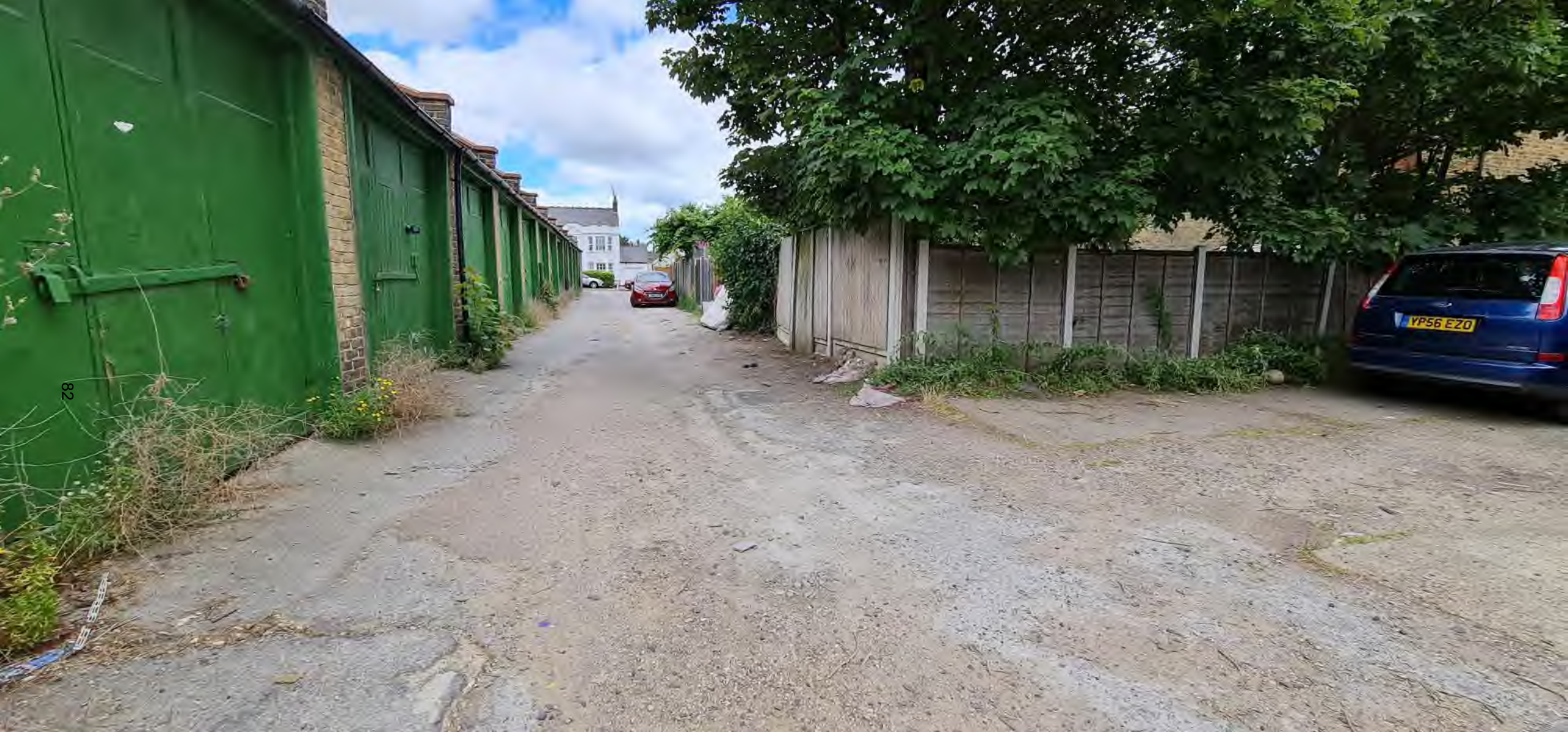
Looking east towards Lovelace Gardens. Application site includes area on the right, to either side of the trees and dividing fence
